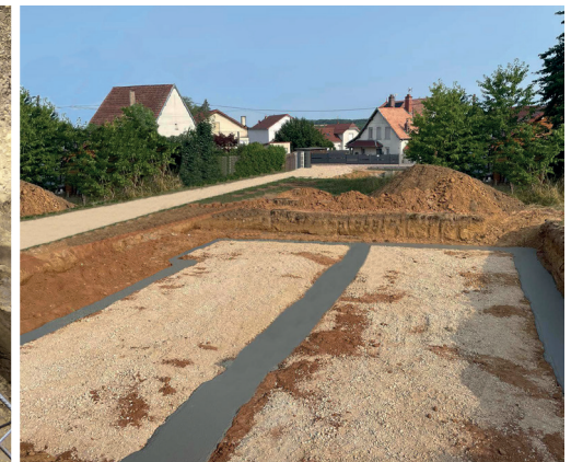
CAST-IN-PLACE FOOTING BEAM
