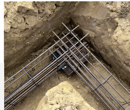
CAST-IN-PLACE FOOTING BEAM
